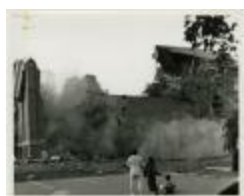
Demolition of Cain Gym (MS 0061-22-12-004)
