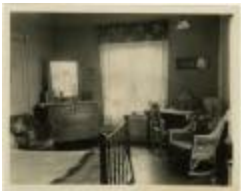
Room in Reid Hall (MS 0061-24-19-010)
