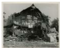
Demolition of Cain Gym (MS 0061-22-12-003)
