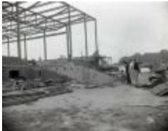
Gym construction and onlookers (MS_0045-250)
