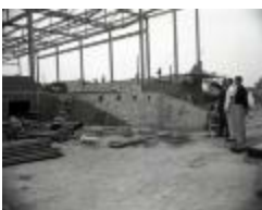
Gym construction (MS_0045-249)
