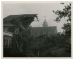
Demolition of Cain Gym (MS 0061-22-12-001)
