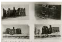
William Smith Hall after the fire of January 1916 (MS 0061-22-13-007)
