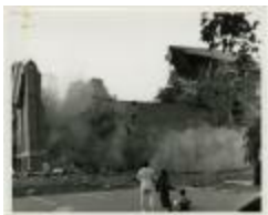
Demolition of Cain Gym (MS 0061-22-12-004)
