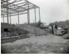
Gym construction and onlookers (MS_0045-250)
