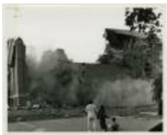
Demolition of Cain Gym (MS 0061-22-12-004)
