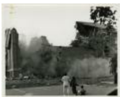
Demolition of Cain Gym (MS 0061-22-12-004) Object identifier: MS 0061-22-12-004 Name: Demolition of Cain Gym
