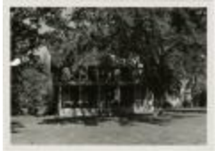
McAlpin House (demolished) (MS 0061-24-13-001)
