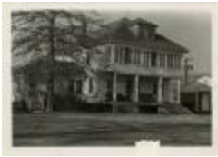
Richmond House (demolished) (MS 0061-25-03-001)
