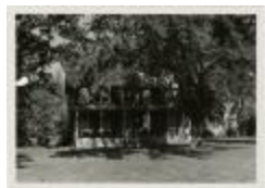
McAlpin House (demolished) (MS 0061-24-13-001)
