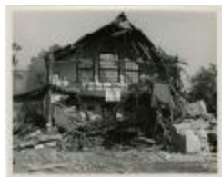
Demolition of Cain Gym (MS 0061-22-12-003)
