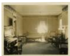
Social Room in Reid Hall (MS 0061-24-19-011)
