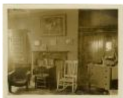
Typical Room in Reid Hall (MS 0061-24-19-012)
