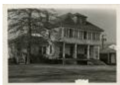
Richmond House (demolished) (MS 0061-25-03-001)
