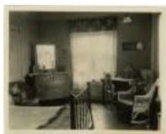
Room in Reid Hall (MS 0061-24-19-010)
