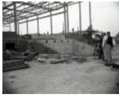
Gym construction (MS_0045-249)
