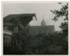
Demolition of Cain Gym (MS 0061-22-12-001)
