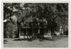
McAlpin House (demolished) (MS 0061-24-13-001)
