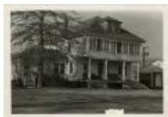
Richmond House (demolished) (MS 0061-25-03-001)
