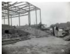
Gym construction and onlookers (MS_0045-250)
