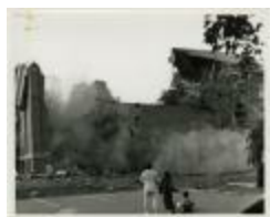
Demolition of Cain Gym (MS 0061-22-12-004)
