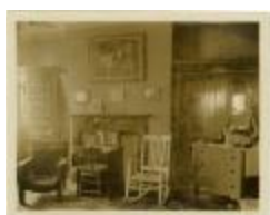
Typical Room in Reid Hall (MS 0061-24-19-012)
