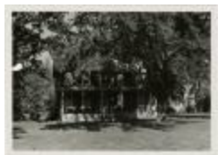
McAlpin House (demolished) (MS 0061-24-13-001)
