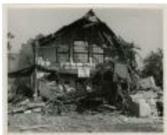
Demolition of Cain Gym (MS 0061-22-12-003) Object identifier: MS 0061-22-12-003 Name: Demolition of Cain Gym
