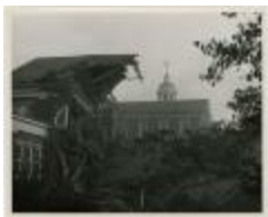
Demolition of Cain Gym (MS 0061-22-12-001) Object identifier: MS 0061-22-12-001 Name: Demolition of Cain Gym
