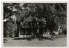
McAlpin House (demolished) (MS 0061-24-13-001) Object identifier: MS 0061-24-13-001 Name: McAlpin House (demolished)
