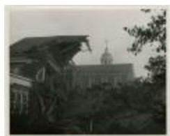
Demolition of Cain Gym (MS 0061-22-12-001)
