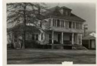
Richmond House (demolished) (MS 0061-25-03-001)
