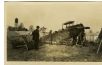
Biplane repairs (MS 0083-01-01-003)
