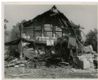
Demolition of Cain Gym (MS 0061-22-12-003)
