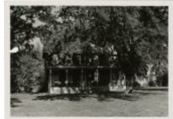
McAlpin House (demolished) (MS 0061-24-13-001)
