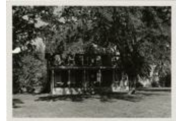
McAlpin House (demolished) (MS 0061-24-13-001)
