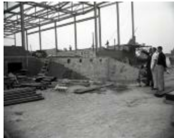
Gym construction (MS_0045-249)
