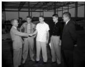
Close-up of men in front of gym construction project (MS_0045-252)
