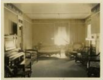
Social Room in Reid Hall (MS 0061-24-19-011)
