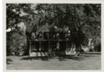
McAlpin House (demolished) (MS 0061-24-13-001)
