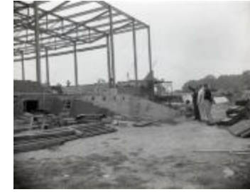
Gym construction and onlookers (MS_0045-250)
