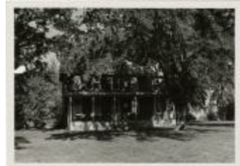
McAlpin House (demolished) (MS 0061-24-13-001)
