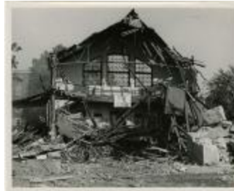
Demolition of Cain Gym (MS 0061-22-12-003)
