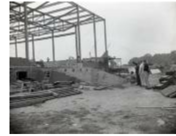
Gym construction and onlookers (MS_0045-250)
