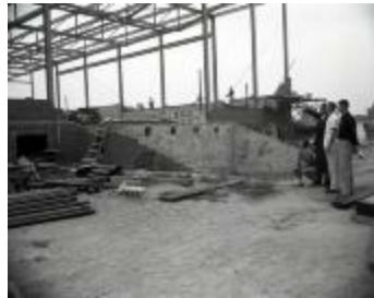
Gym construction (MS_0045-249)
