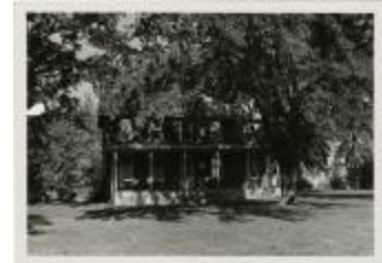
McAlpin House (demolished) (MS 0061-24-13-001)
