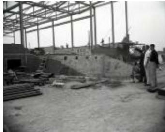
Gym construction (MS_0045-249)
