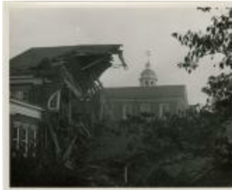
Demolition of Cain Gym (MS 0061-22-12-001)
