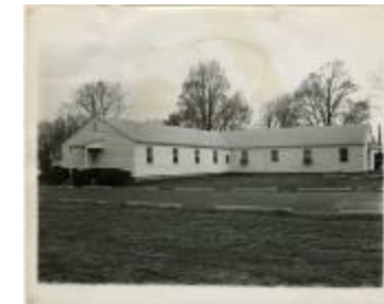
G.I. dorms (demolished) (MS 0061-23-16-007)
