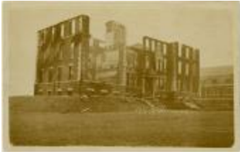
Ruin of William Smith Hall after the fire in 1916. (MS 0061-22-13-001)
