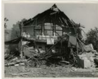
Demolition of Cain Gym (MS 0061-22-12-003)
