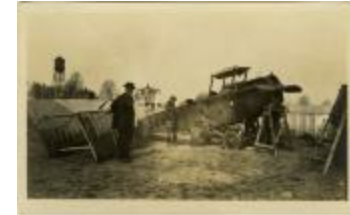
Biplane repairs (MS 0083-01-01-003)
