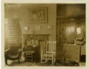
Typical Room in Reid Hall (MS 0061-24-19-012)
