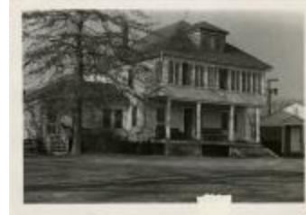
Richmond House (demolished) (MS 0061-25-03-001)
