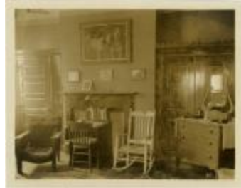
Typical Room in Reid Hall (MS 0061-24-19-012)
