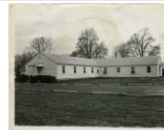
G.I. dorms (demolished) (MS 0061-23-16-007)
