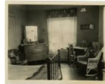
Room in Reid Hall (MS 0061-24-19-010)
