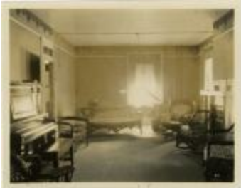
Social Room in Reid Hall (MS 0061-24-19-011)
