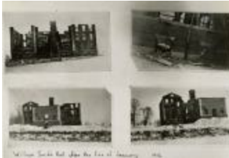
William Smith Hall after the fire of January 1916 (MS 0061-22-13-007)
