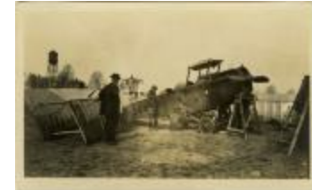
Biplane repairs (MS 0083-01-01-003)
