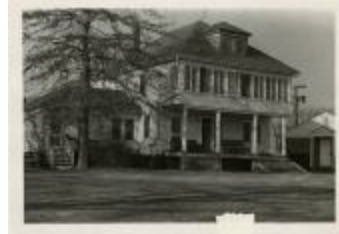
Richmond House (demolished) (MS 0061-25-03-001)
