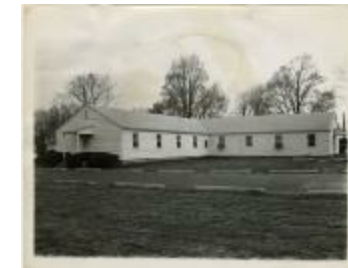
G.I. dorms (demolished) (MS 0061-23-16-007)
