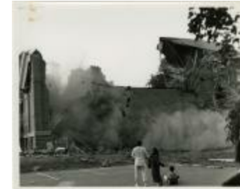
Demolition of Cain Gym (MS 0061-22-12-004)
