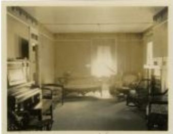
Social Room in Reid Hall (MS 0061-24-19-011)
