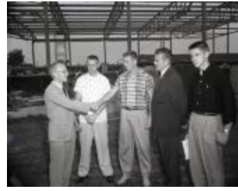
Group of men in front of gym construction (MS_0045-251)
