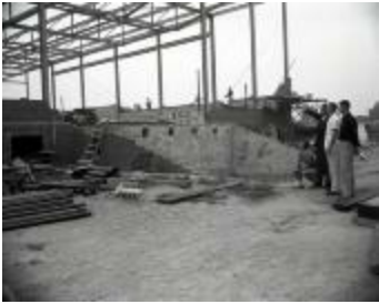
Gym construction (MS_0045-249)
