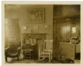
Typical Room in Reid Hall (MS 0061-24-19-012)
