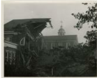
Demolition of Cain Gym (MS 0061-22-12-001)
