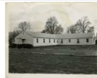
G.I. dorms (demolished) (MS 0061-23-16-007)
