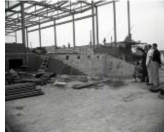
Gym construction (MS_0045-249)
