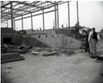
Gym construction (MS_0045-249)
