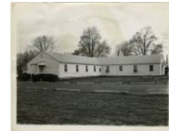
G.I. dorms (demolished) (MS 0061-23-16-007)
