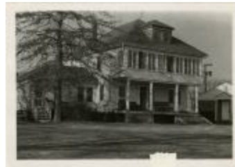
Richmond House (demolished) (MS 0061-25-03-001)
