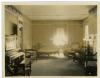
Social Room in Reid Hall (MS 0061-24-19-011)
