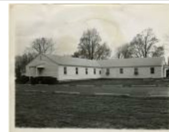
G.I. dorms (demolished) (MS 0061-23-16-007)
